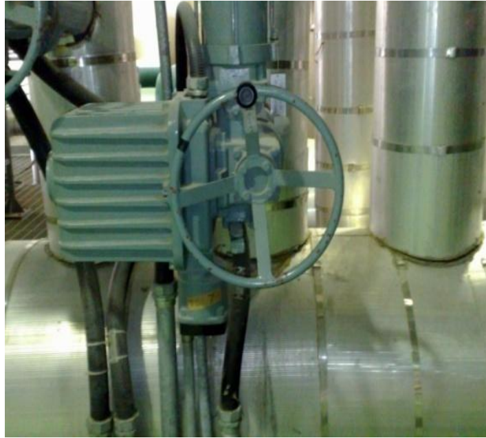
Figure 3.20 Between two noise source X17 and X19, (STU1)
