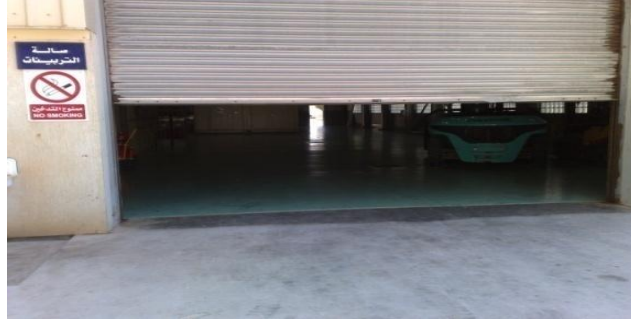
Figure 3.4 at the door of unit,( STU3)
