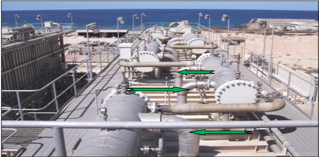
Figure3.11 The pre-heaters of Zawia MED Power Plant[29]
