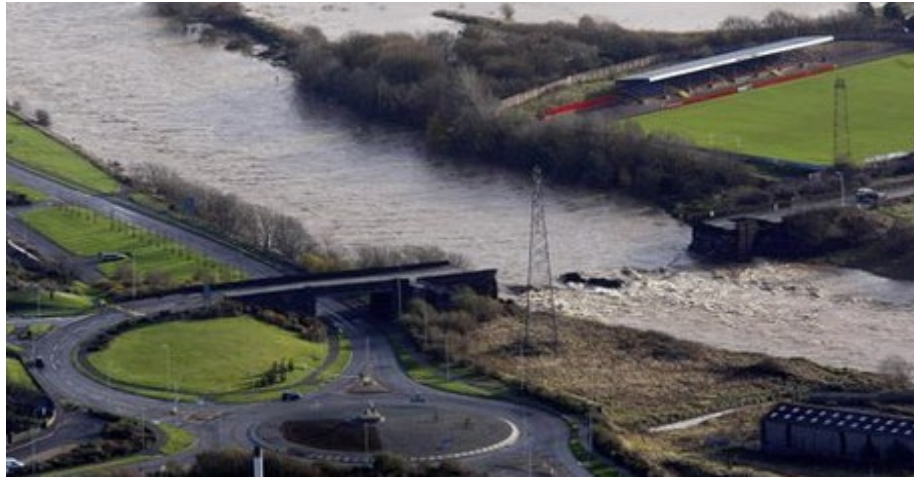
Figure 1-1: Workington's Northside Bridge (BBC News, 2016b).
